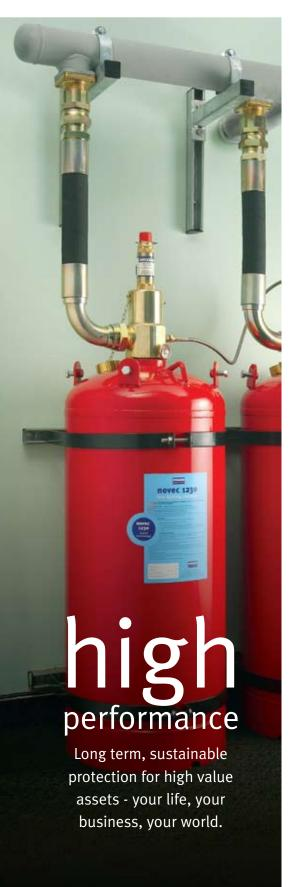
Hygood Sapphire™ Systems, using 3M™ Novec™ 1230 Fire Protection Fluid have emerged as the solution of choice for fire extinguishing systems to protect high value assets and processes. Sapphire is a clean agent system which is proven to be environmentally friendly.
